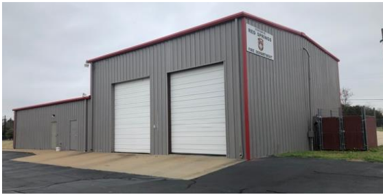
Figure 131: Red Springs VFD, Station 2
